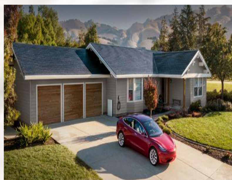
Solar panel tiles on roof
